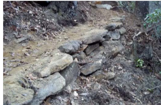
Rock Retaining Wall
